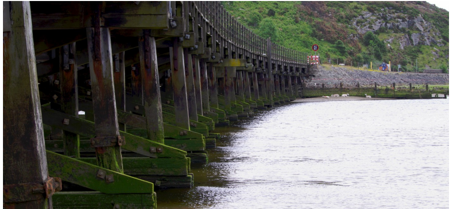
Illustration 1: Pont Briwet (Existing Structure)
