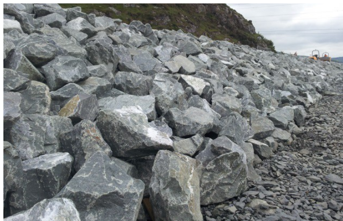
Illustration 3: Rock Armour Protection to embankments
