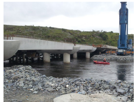
Illustration 2: New bridge structure (Under construction)
