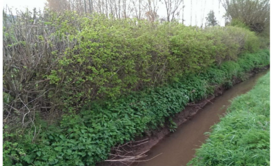
Illustration 1: Hedgerow on informal defence at Five Bridges
