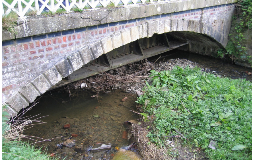
Illustration 1: Lledan Brook Aqueduct
